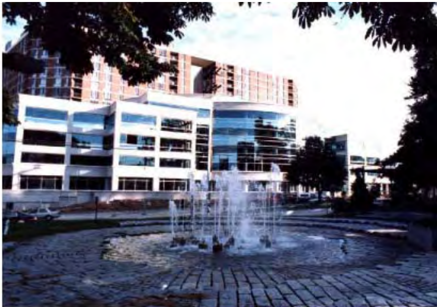
CHK Office HQ Bldg, Silver Spring, MD. (a/CHK)
